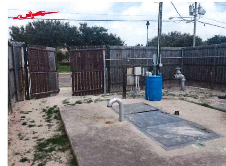
2 EXISTING INTERIOR CONDITIONS N.T.S.
